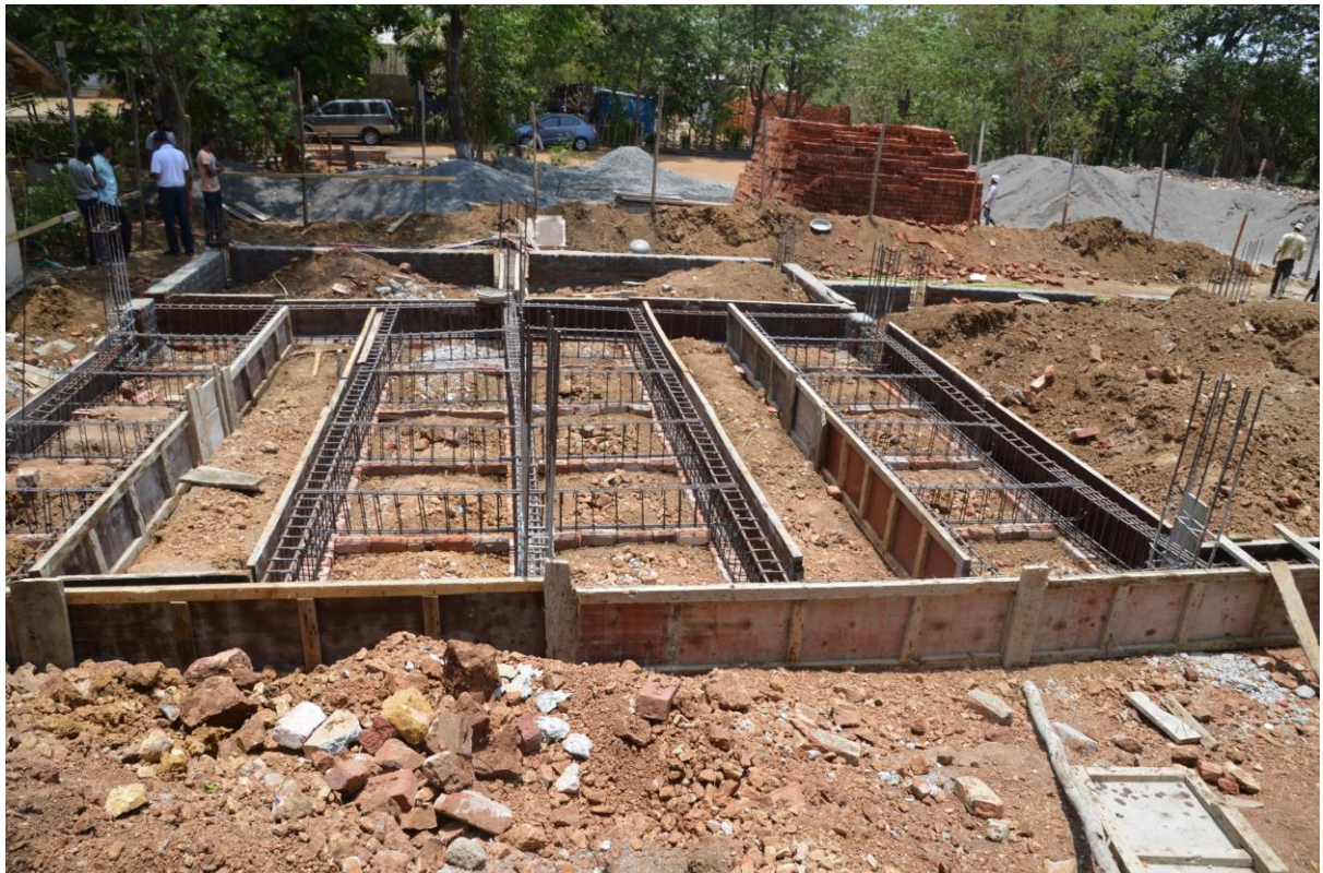
CASTING OF GROUND BEAMS
