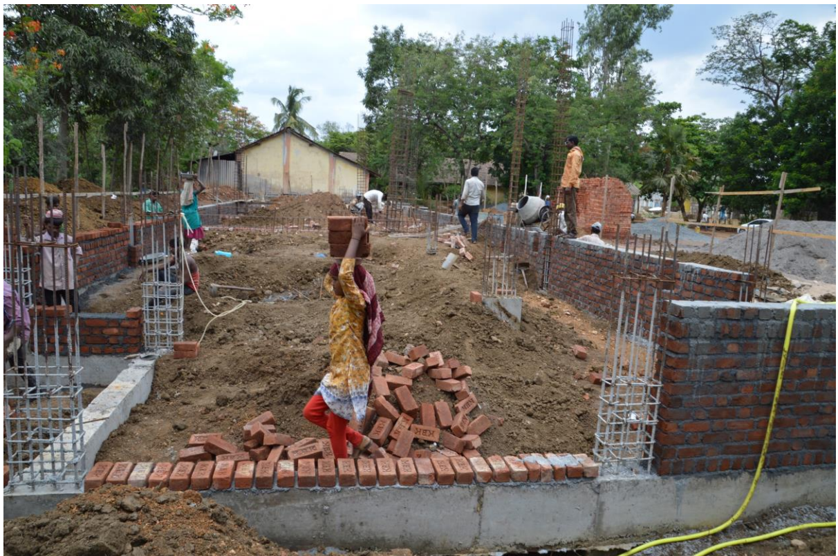
BRICK MASONRY FOR PLINTH
