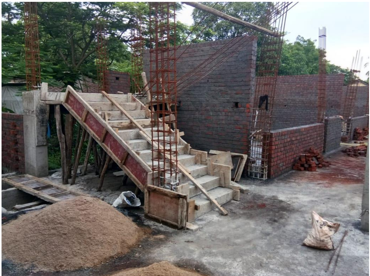
BRICK WORK FOR GROUND FLOOR
