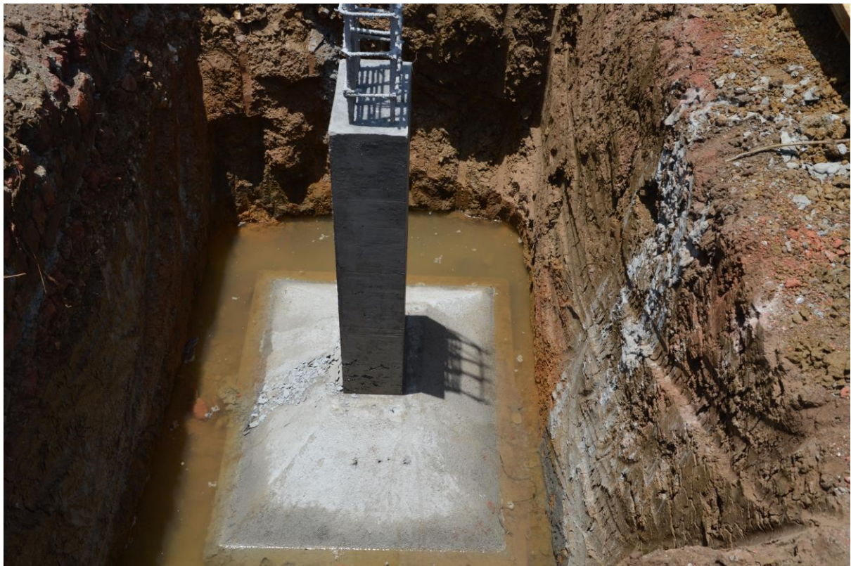
CASTING OF FOUNDATION
